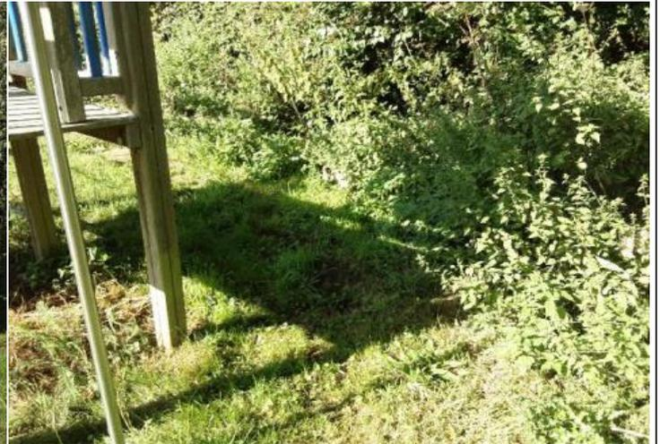
**Finding:** The hedge forms a hard object within the falling space of the equipment and there is also insufficient surfacing provided in contravention of BS EN 1176 Part 1
