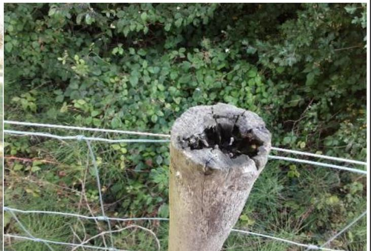
**Finding:** There are areas or parts of the timber on the structure that have rotted
