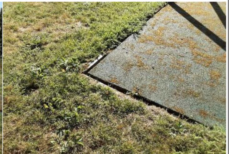
**Finding:** The surface is lifting at the edges and creating trip points
