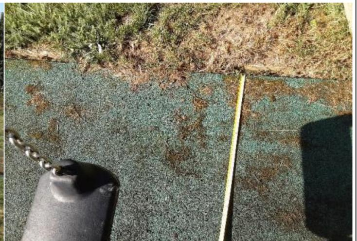
**Finding:** The surfacing width under each seat is less than 1.75 metres and fails the requirements of BS EN 1176 Part 2
